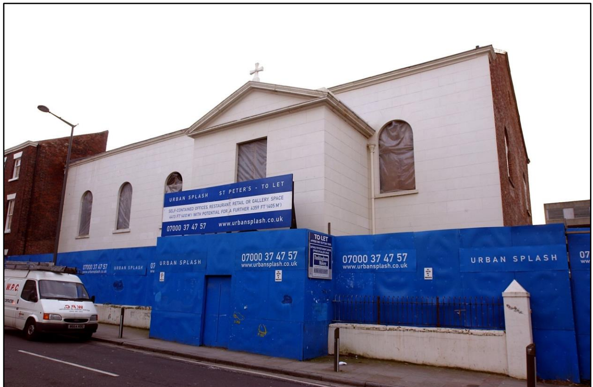
St Peter's Church Seel Street Liverpool which is to be converted into offices by developer urban splash in 2003 – Above images - Copyright Liverpool Echo
