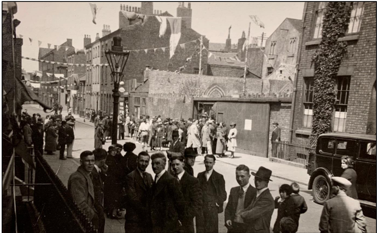
A view of Seel Street in 1938 showing the St Peter's Gardens and 55 Seel Street on the right hand side of the street. This is showing the 150 th Anniversary celebrations of the Church. Copyright Liverpool Record Office.
