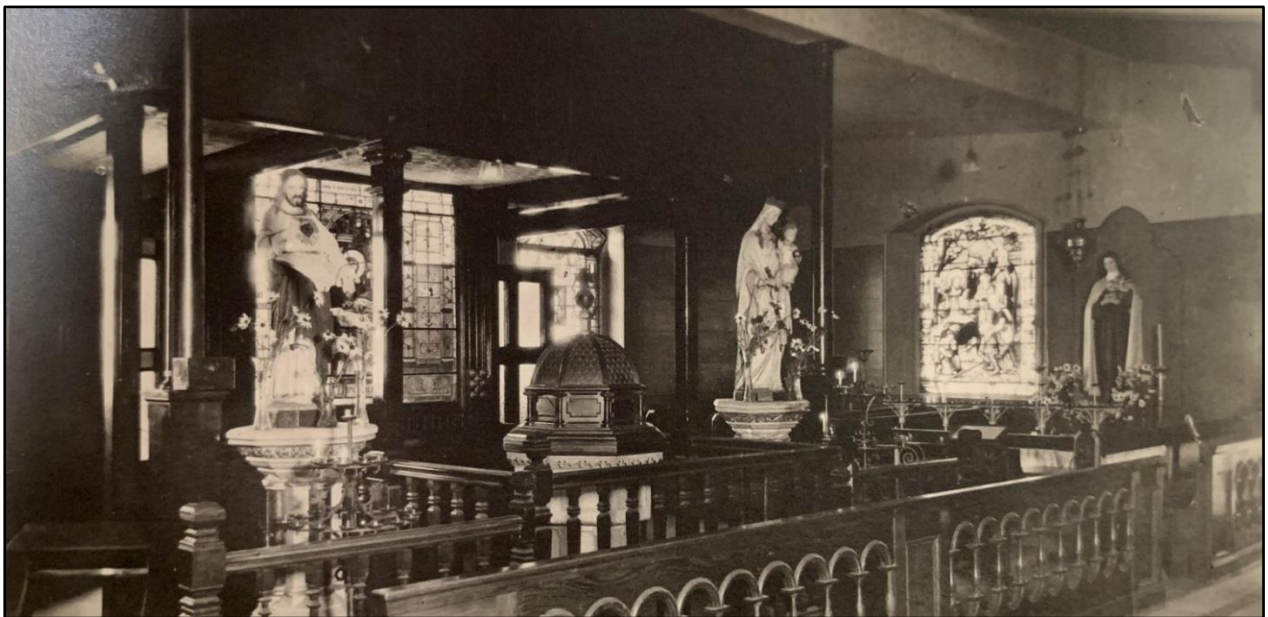
Interior of the Church – Copyright Liverpool Record Office
