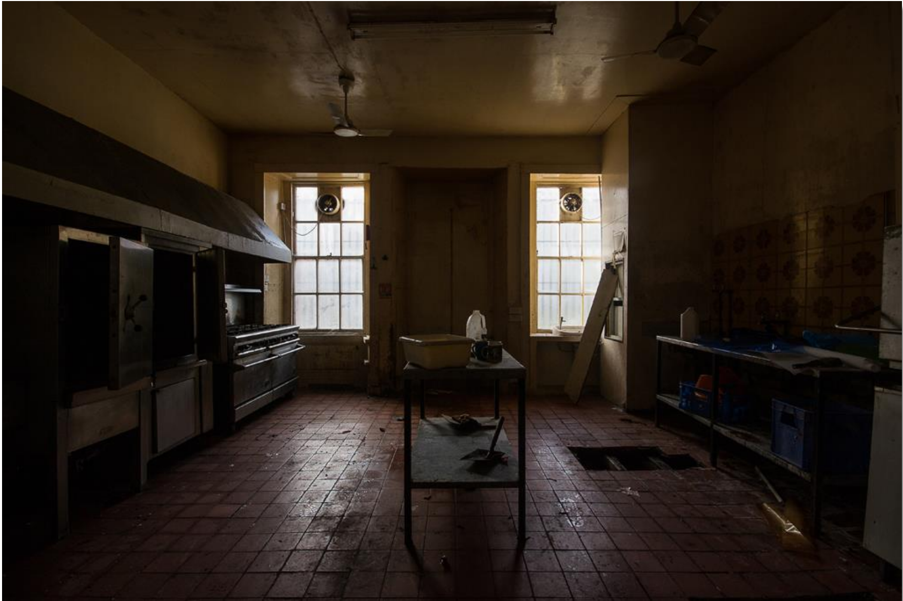
7. Viewing the kitchen area – the floor has rotted on the right-hand side.
